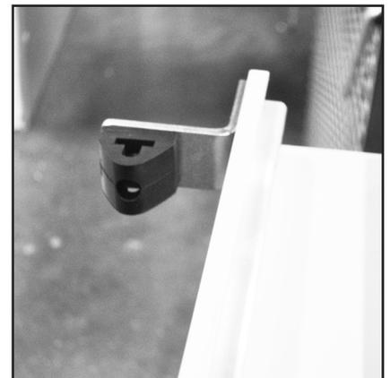
The **Floor Roller** keeps the door from swinging away from the wall, and presses the gasket against the wall when the door is closed. Position the base as shown (*Fig. 7*) and bolt to the floor. The angled plate in the sketch is already attached to the door.
